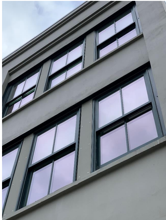
Rehabilitated Upper Storey Facade
