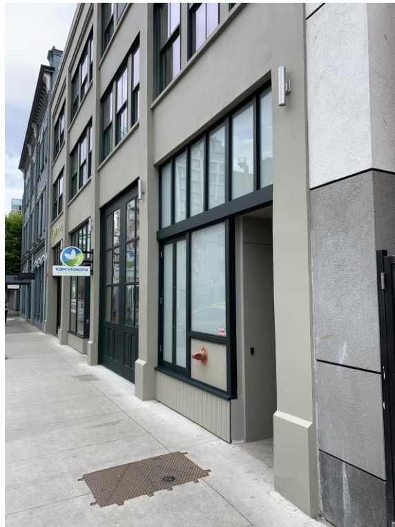
Rehabilitated Ground Floor
