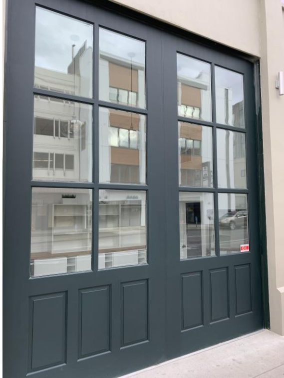
Rehabilitated Stable Doors
