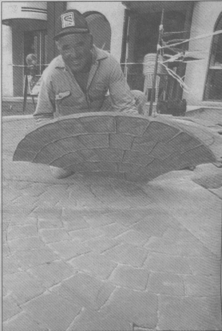
■ BASTION SQUARE gets a new look as part of restoration program. Although this looks like brick, it's phoney — created with a mould which is being employed by city worker Ivano Chelini.
