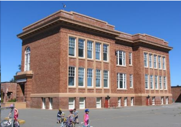
Oaklands School- 2827 Belmont Avenue (1913 wing)- Register Status
