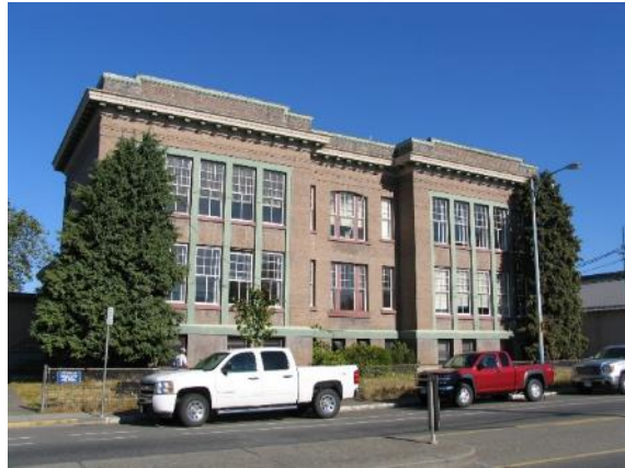
Burnside School- 3130 Jutland Road (1913 wing)
