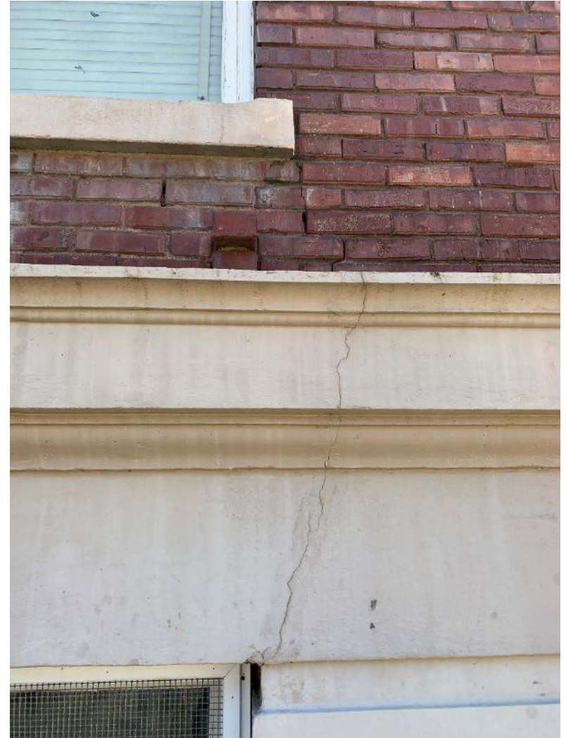
Spider crack in foundation
