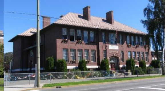
Quadra School and Annex- 3031 Quadra Street (1914 wing and annex)
