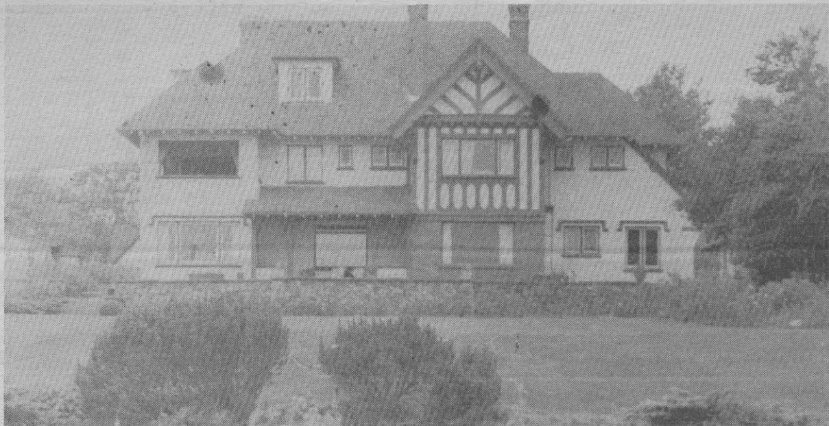
The Pendray Estate property, shortly to be subdivided. The home will remain and Council is endeavouring to control the development of the land (see Council News).
