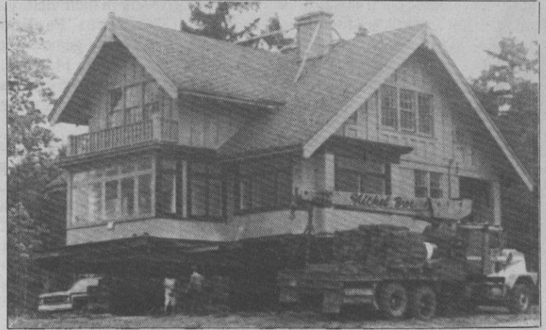
HERITAGE LOST out in Oak Bay two years ago when this house at 2425 Oak Bay Ave. was moved from its foundation and barged to Yellow Point, as was the house shown on opposite page at 2551 Beach Dr. The building, dating back to 1910, was slated for demolition. Both houses were bought for a dollar by John Mathers.
