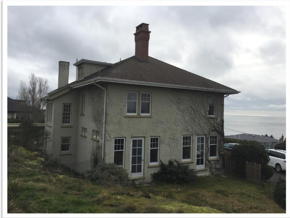
644 Beach Drive: west exposure
