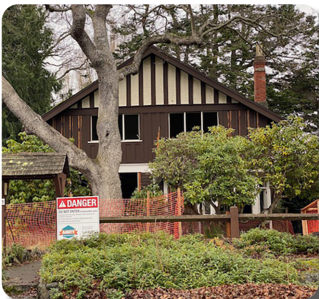
785 Island Road. top, file photo; bottom, December 2020.
