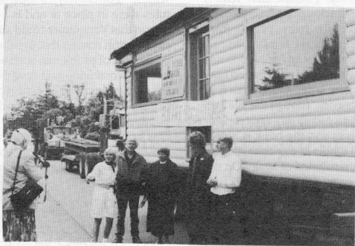
The Emily Carr cottage ready for moving. Roger Tallentire photo.
