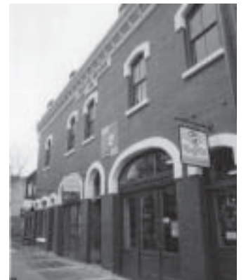
Hart Block City of Victoria photograph
