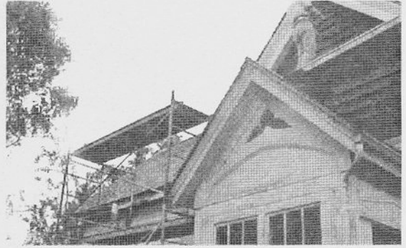
Careful removal of 1950s siding
