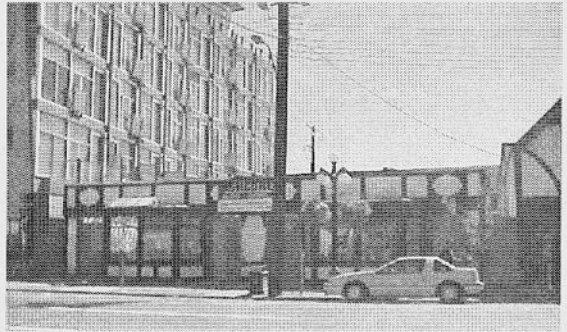
The Chelsea Block prior to demolition.
