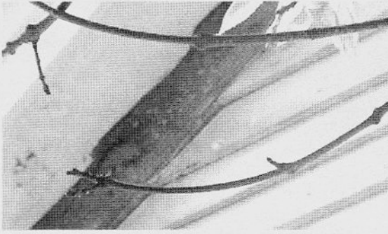
Removal of 1950s siding reveals original material beneath
