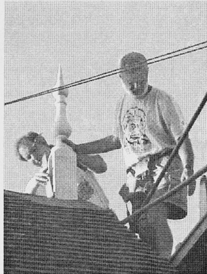
The first finial is set in place
