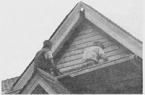
Workers on the west side gable
