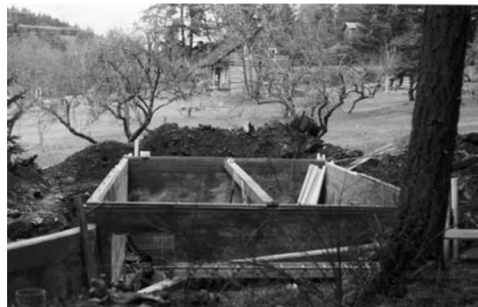
New foundation February 4, 2001 Note Caleb Pike Homestead in background
