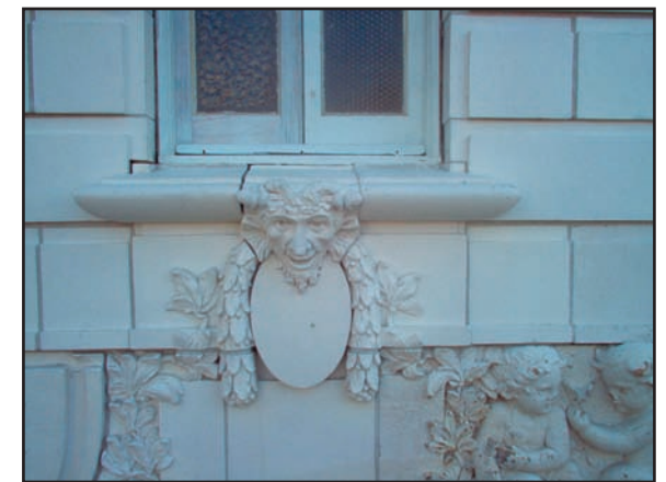
Newly sculpted noses to repair damage
