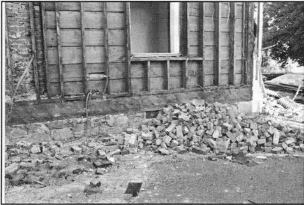
Discarded bricks. July 31, 2006
