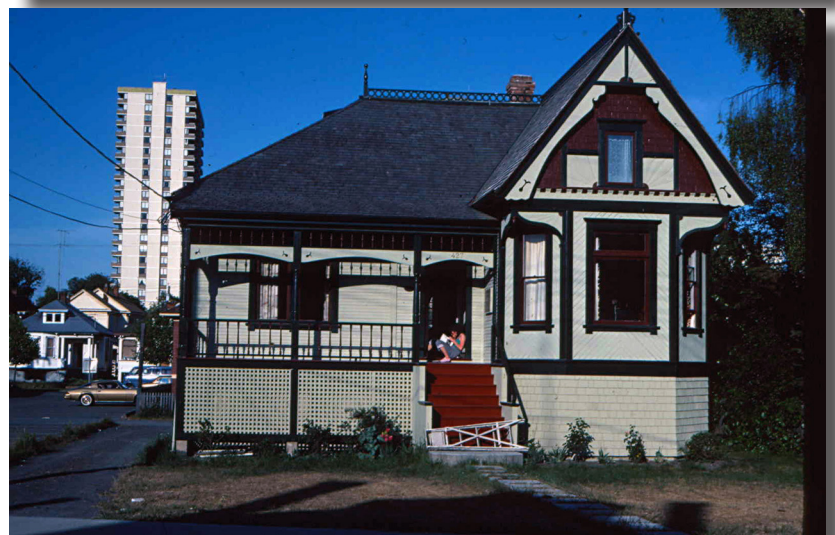
The Jackson House just after moving and later as restored.
