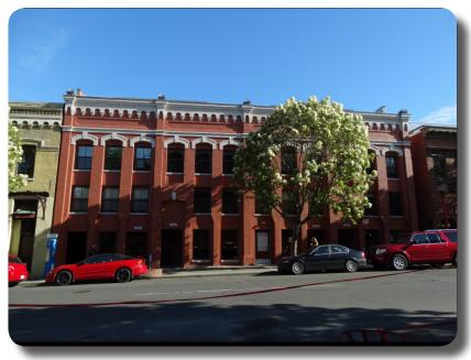
Exterior brick masonry was re-built to the original designs with extensive repairs and repointing being carried out.
