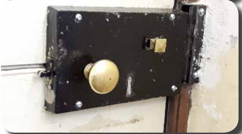
Top: rotten wood; bottom: broken door lock. Both photos by Ken Johnson
